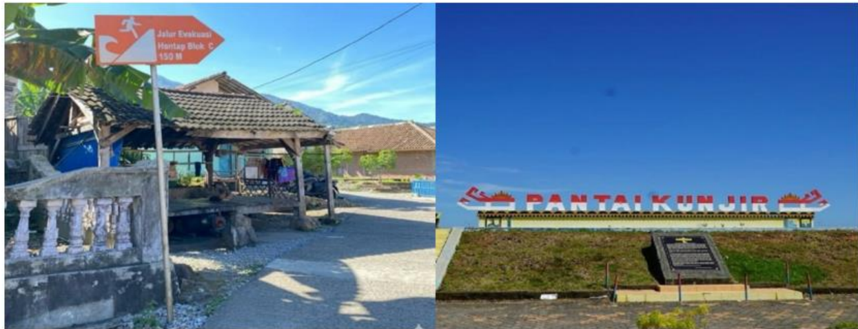
Figure 7. Tsunami evacuation route signage and breakwater in the study area
