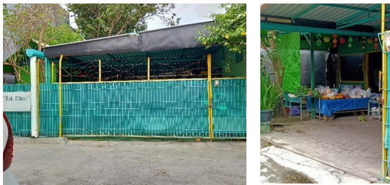
Figure 5. The forming of social spaces in Prawirotaman: space negotiation (left: the closing of a transition area became a private terrace, right: the opening of a transition area became a temporal tavern)
