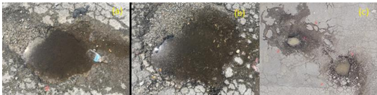
Figure 3. (a) Potholes A (b) pothole B and (c) aerial image for both potholes.
