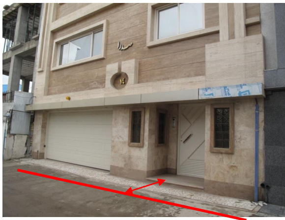
Figure 8: Design plan of stop place as a transition place outside the house
